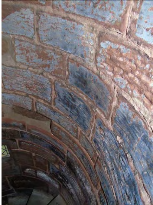
Interior of spiral staircase. Note moisture to masonry face.
