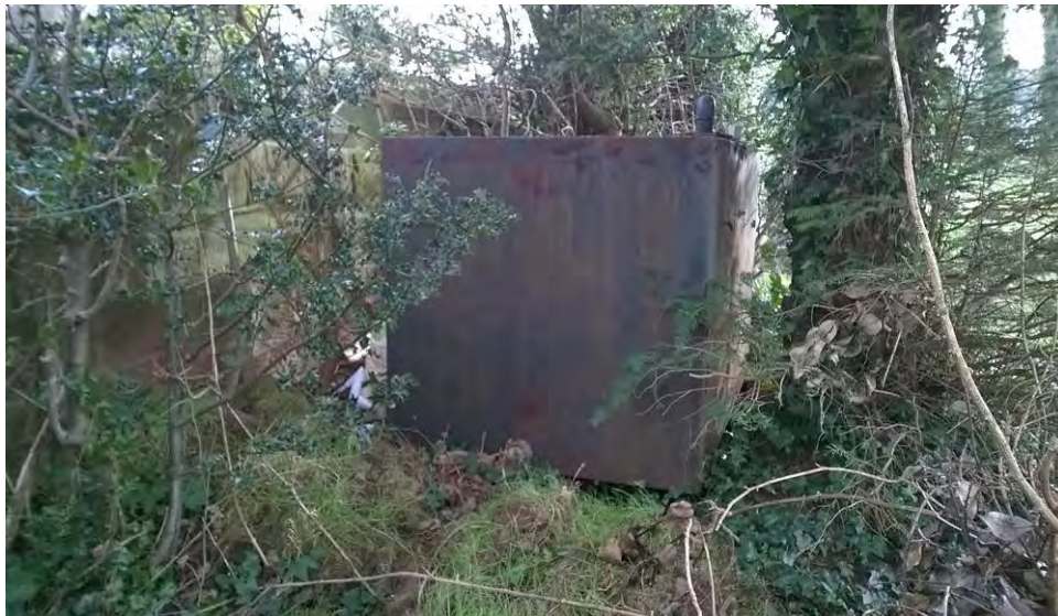
The oil tank.
