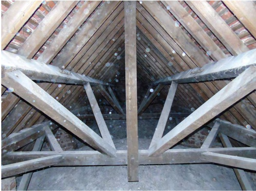
Nave roof space. General photograph.
