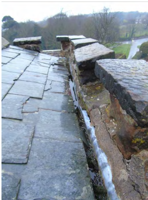
Roof and parapet gutter to the Old Tower.
