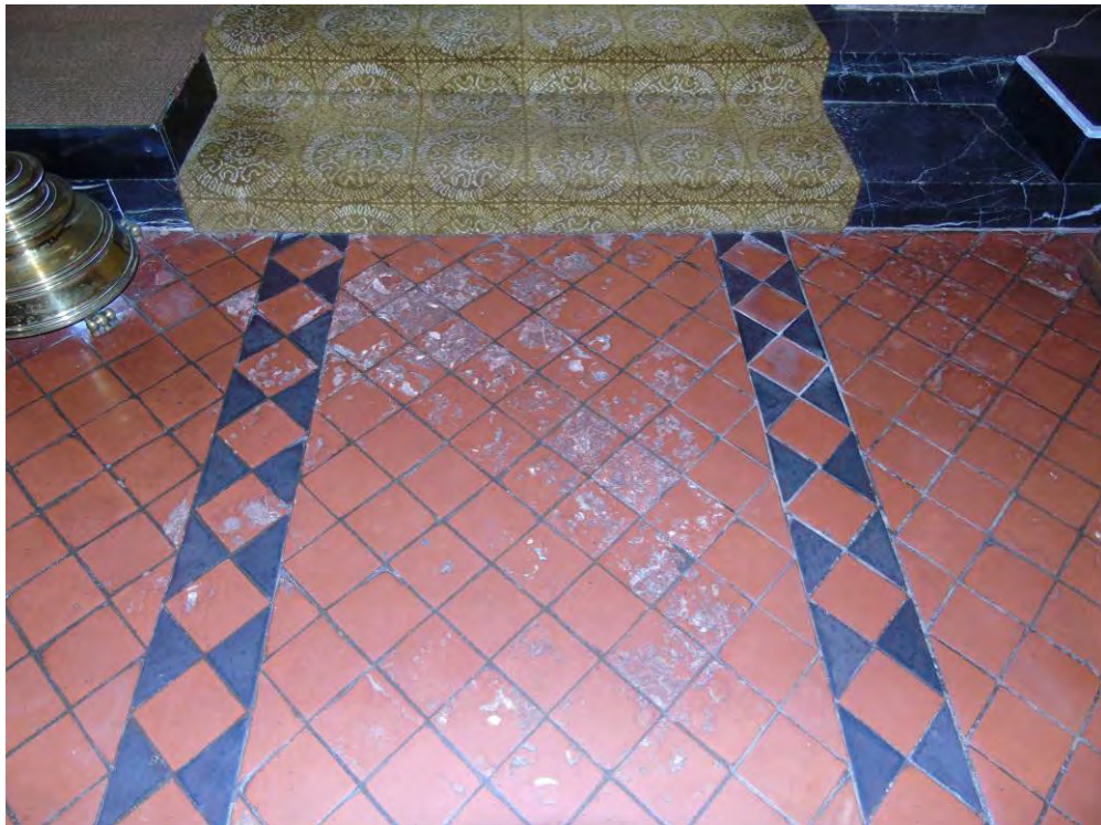
Damaged floor tiles within nave.
