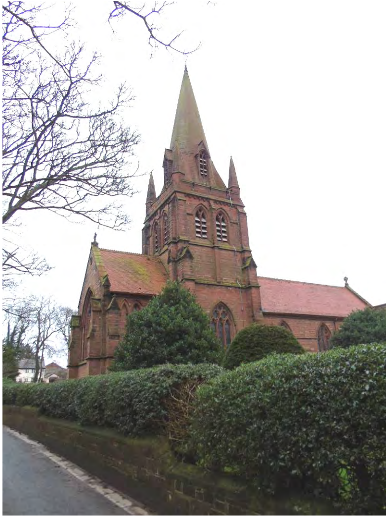
View from North East
