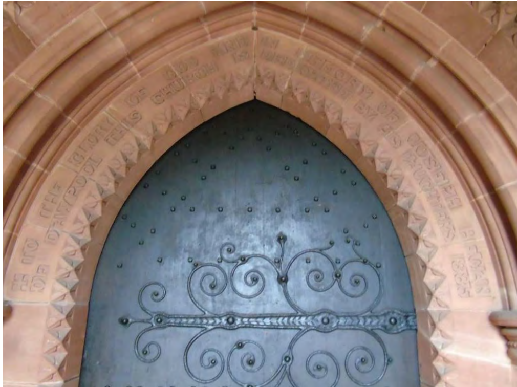
North porch door and opening.
