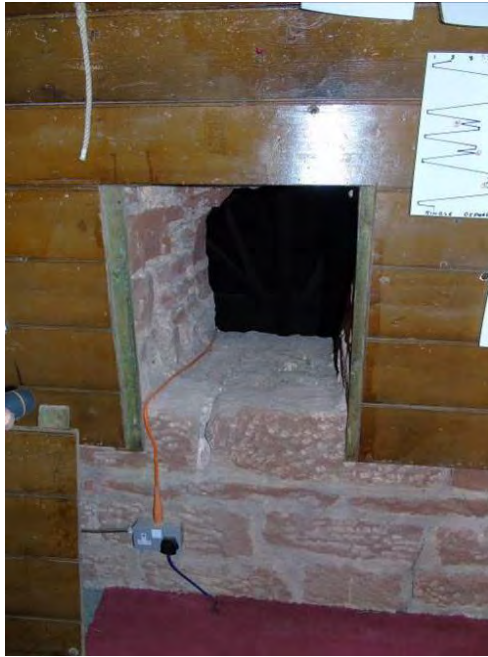
Roughly formed opening into nave roof void.
