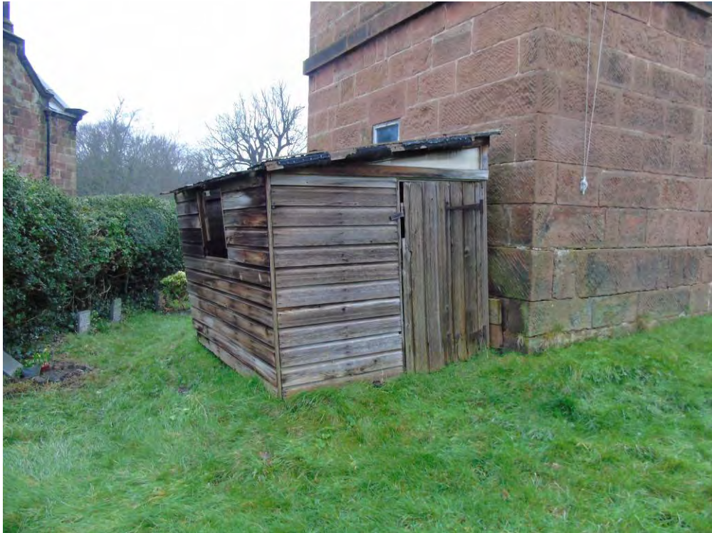
Dilapidated shed abutting the Old Tower.
