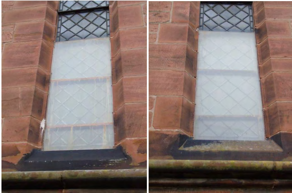
Polycarbonate window protection. Note corroding saddles bars.
