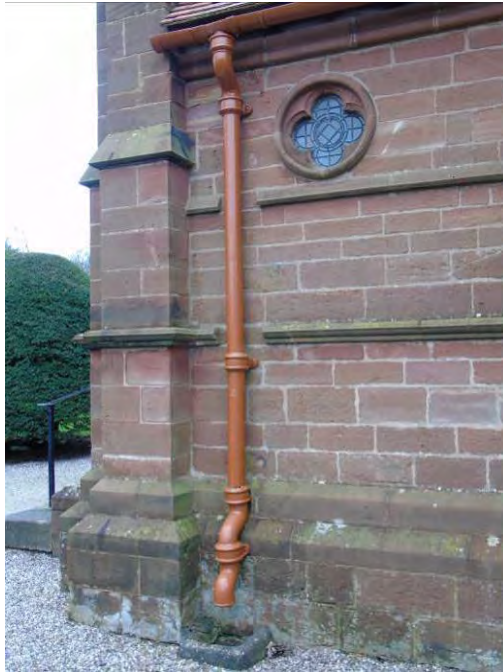
North porch west downpipe.
