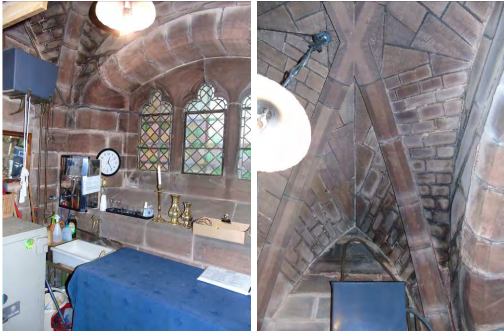
Water damage within vestry.
