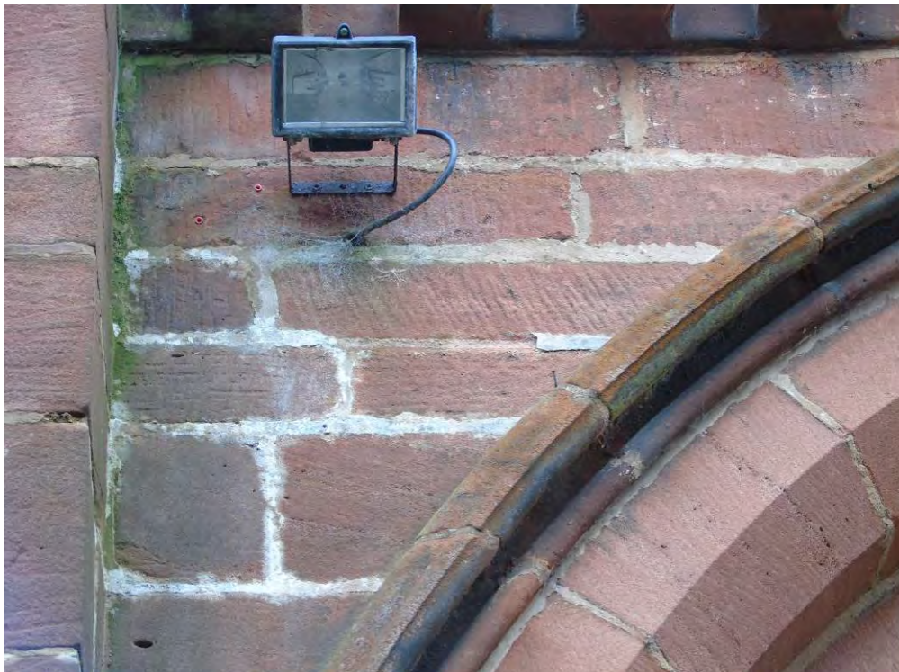
Detail of shallow cement pointing that is failing.
