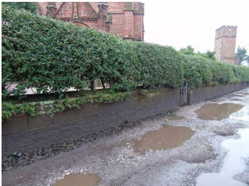
Vegetation growth to west boundary wall.
