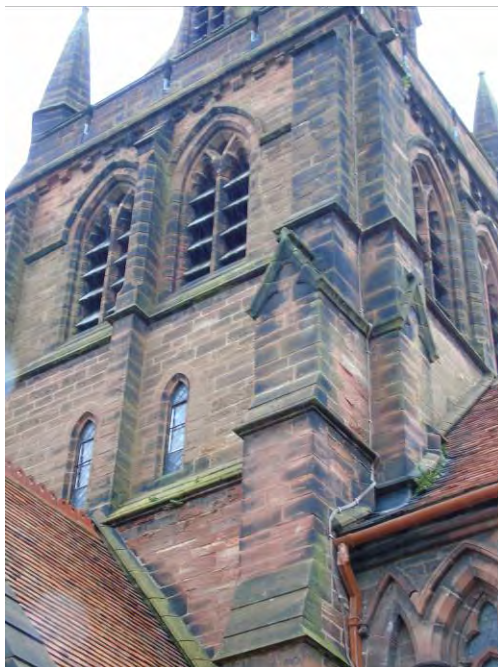
South elevation of tower. Note vegetation growth beneath lancet windows.
