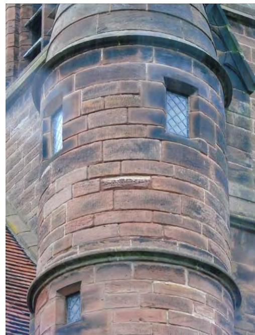
Open mortar joints and wind erosion to spiral stair.
