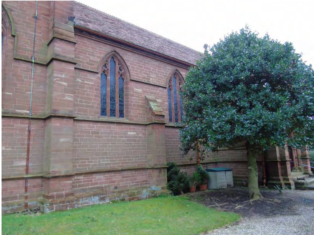
Nave North Elevation
