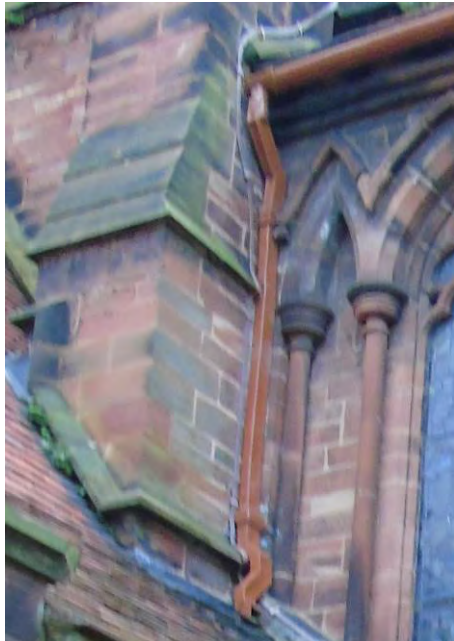
Detail of south sanctuary downpipe.
