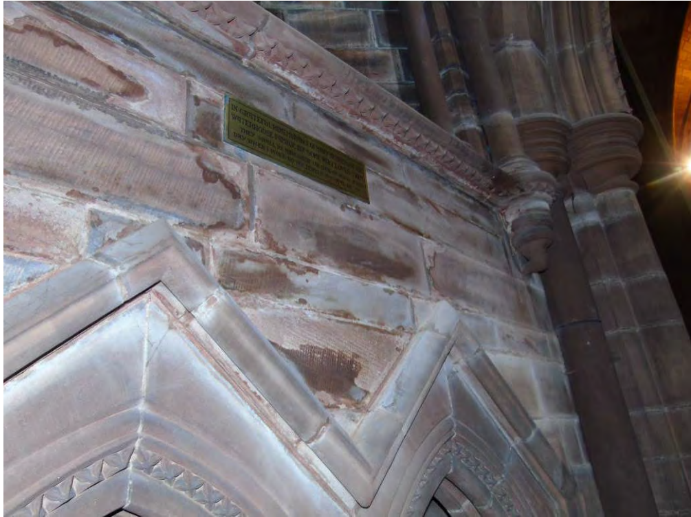
Detail of water damage within sanctuary.
