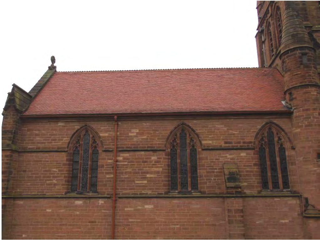
Nave south pitch. General photograph.
