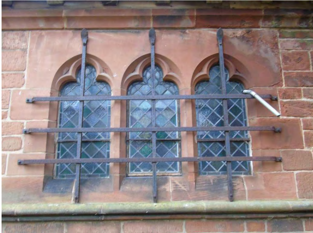
East windows to vestry. Note corrosion to iron bars / grille.
