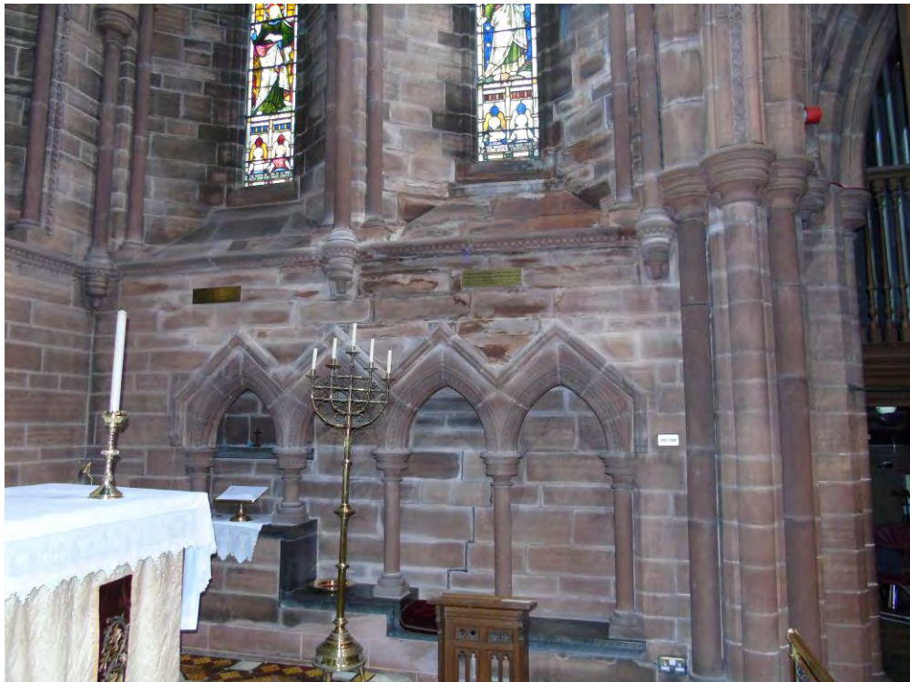
Water damage within sanctuary.
