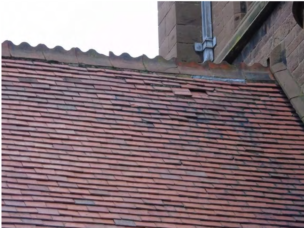
Nave south pitch. Detail of abutment to tower.
