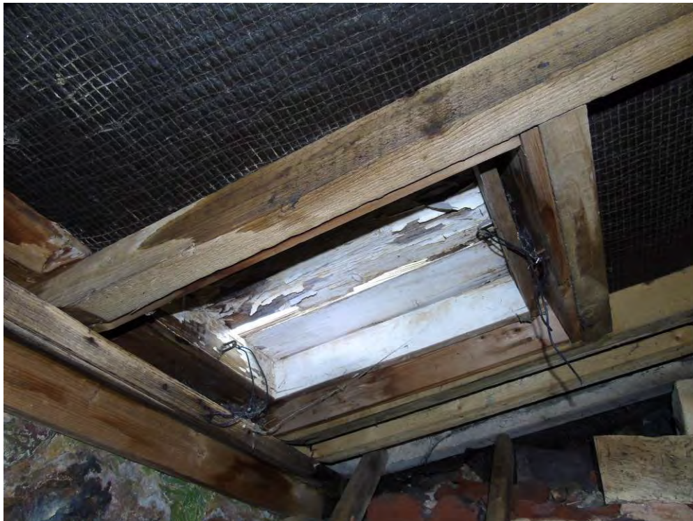
Roof access hatch decayed.
