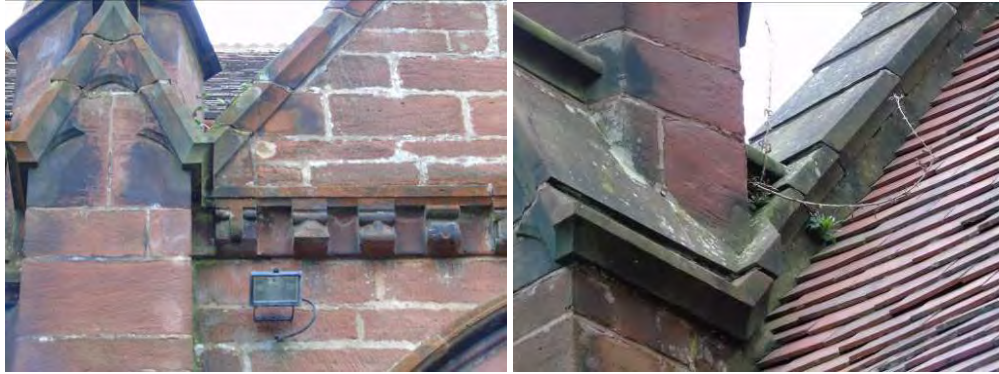
Vegetation growth to copings. / cement flashing to north porch.
