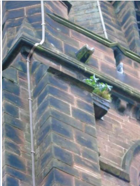
Blocked hopper to tower.
