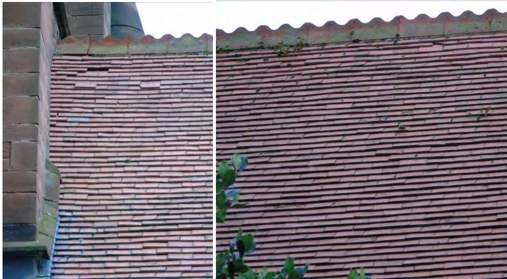
Nave north pitch details.
