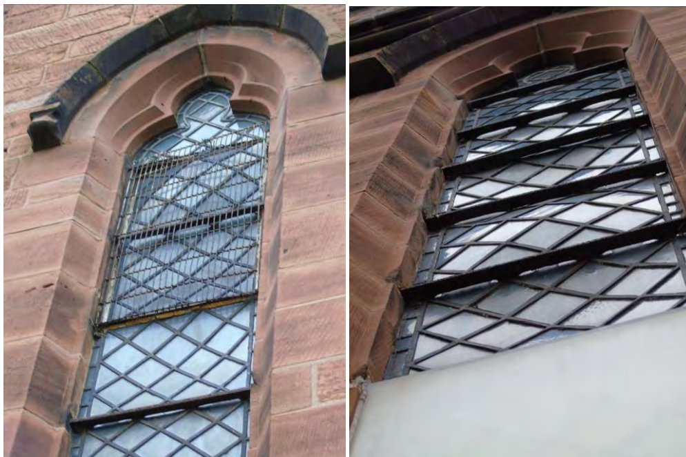
Corroding metal casement and distorted glass.
