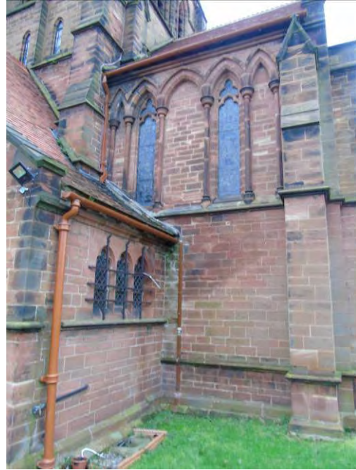
Chancel south elevation. Note water saturated masonry and vegetation growth.
