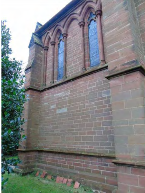
Chancel north elevation.
