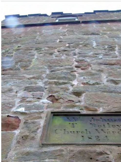
Cement pointed movement crack.
