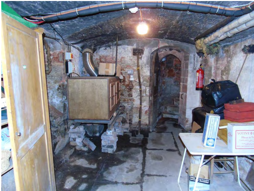
The heating chamber. Note piers to organ blower.
