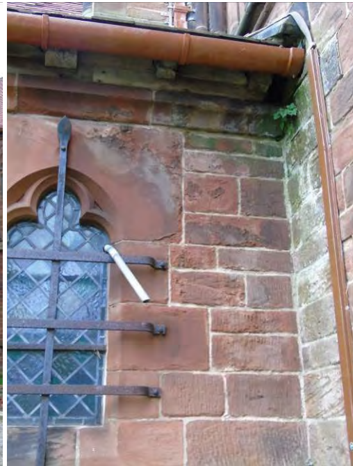
Vestry, east elevation. Water saturated masonry.
