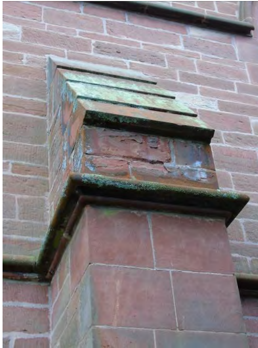
Erosion to central buttress. Note cement pointing.
