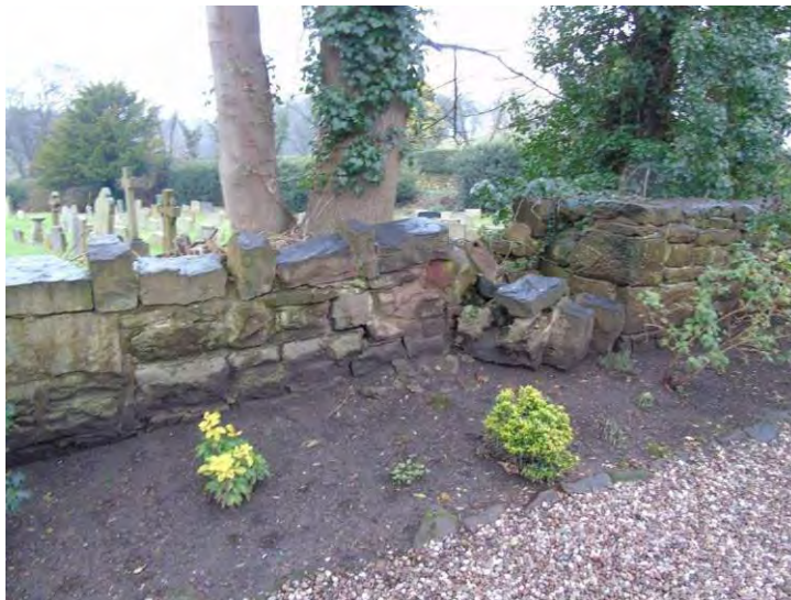
Collapsed section of low south boundary wall.
