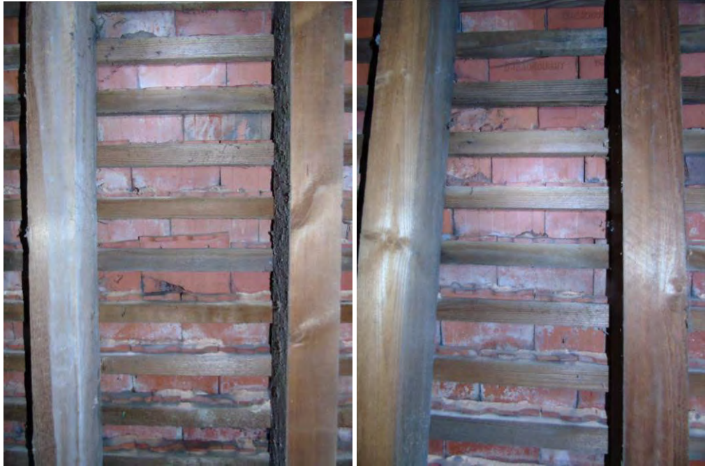
Details of cracked, displaced and replacement tiles.
